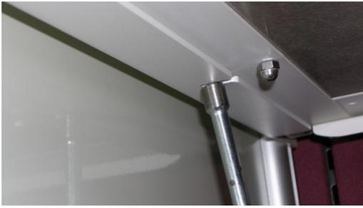
NOTE: The nut driver can mark the paint.
